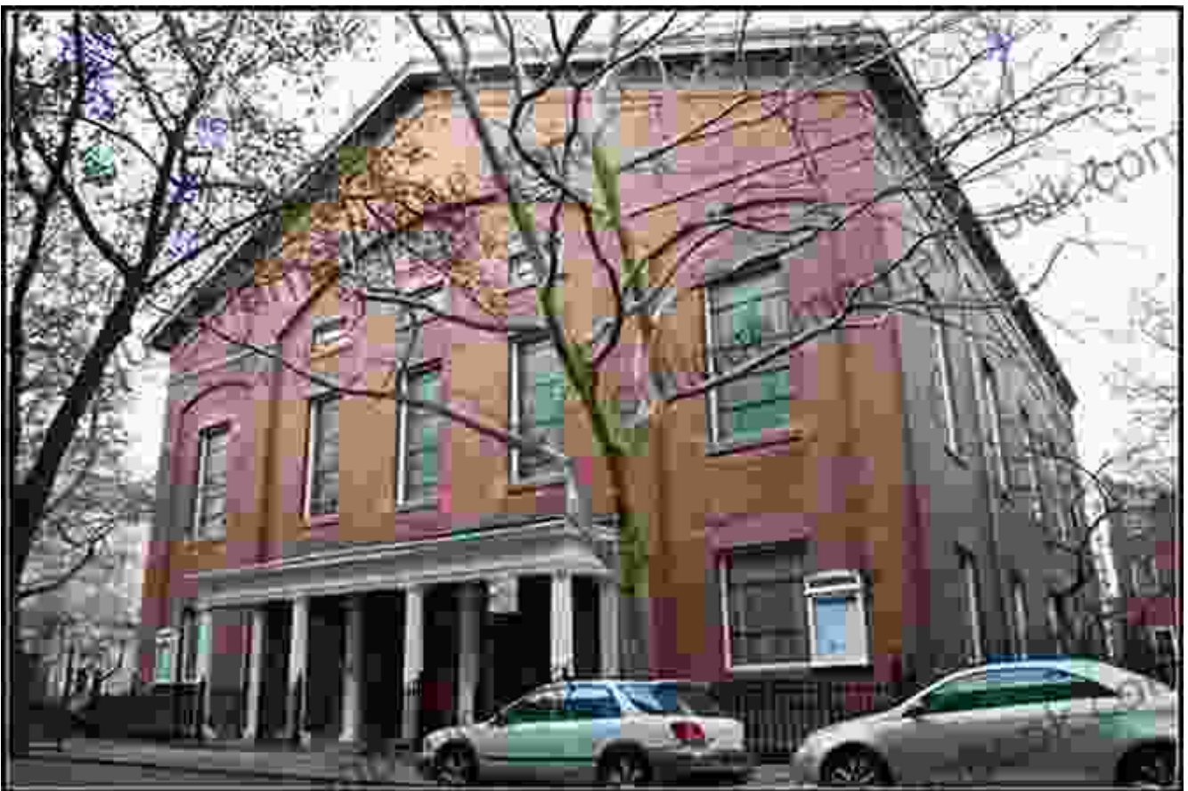
The Gothic Revival Plymouth Church in Brooklyn Heights, built during the Victorian era.
